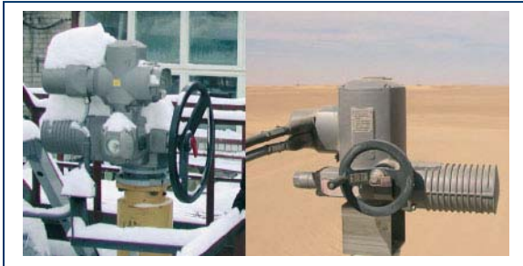
Electric actuators automate industrial valves in the energy, chemical, waste water, and other industries
